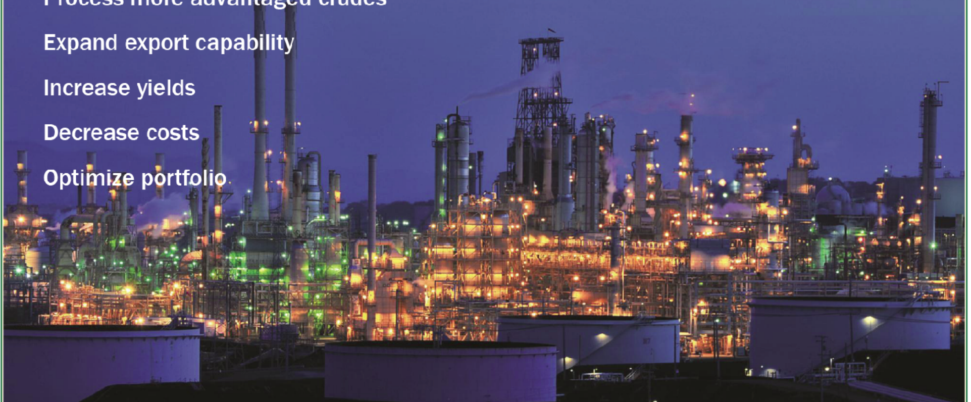
San Francisco Refinery, Rodeo Facility. San Francisco, California.
