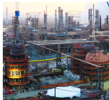
Chevron Richmond's FCCU, during major repairs
