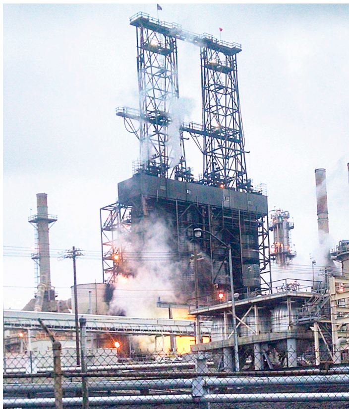
Delayed Coker, Phillips 66 Refinery, Rodeo, CA
