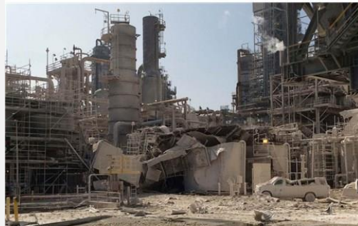
ExxonMobil Torrance 2014 Explosion : Workers were luckily away from the explosion. U.S. Chemical Safety Board found a vessel containing deadly Hydrogen Fluoride, could have been catastrophically destroyed.
