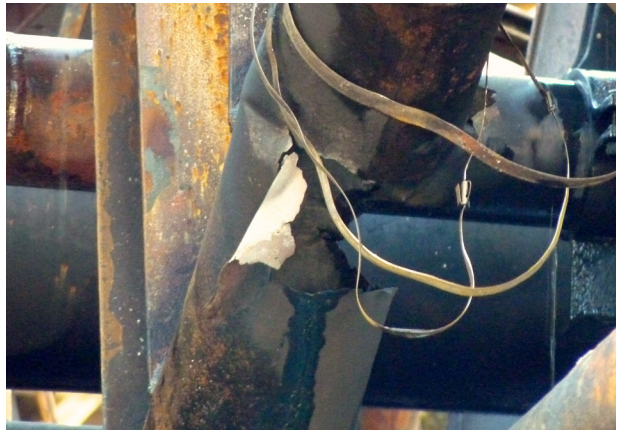
Figure 1. The pipe rupture involved in the 6 August Richmond crude unit fire. Photo CSB.
