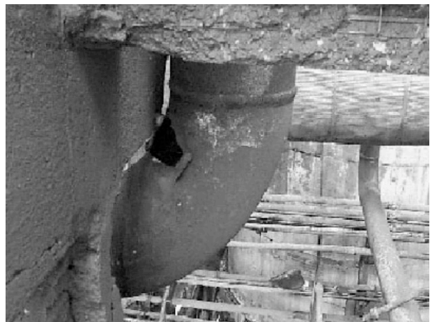
Figure 2. Sulfidation corrosion failure of a pipe elbow at another refinery. Photo API (2003).
